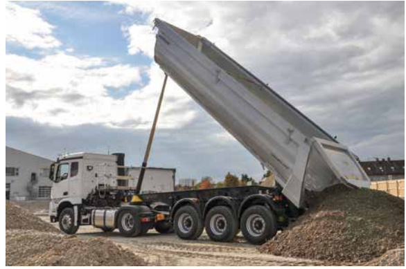
... to the construction site
